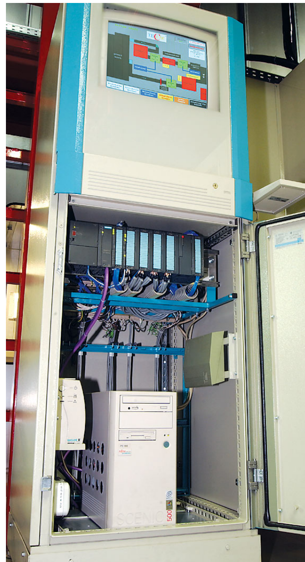
Safe and reliable: higher-level Simatic WinAC station with software PLC and UPS
