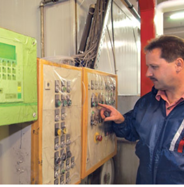
To enable operator control and monitoring on site, a number of Simatic Operator Panels are connected to the WinAC controllers
